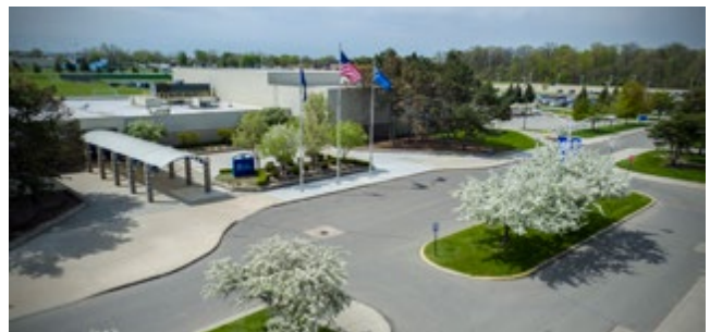
Guest drop-off zone at the main entrance meets a covered walkway in case of inclement weather, and can also be staged as an outdoor exhibit area for special vehicles or event services.
